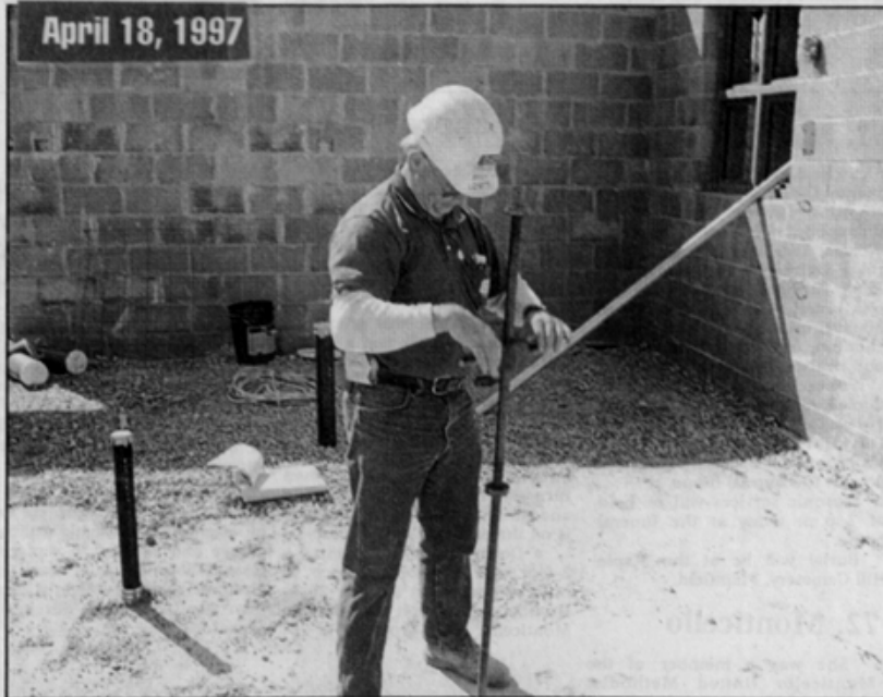
Bill Lovitt of Environmental Testing Services checks density of ground
